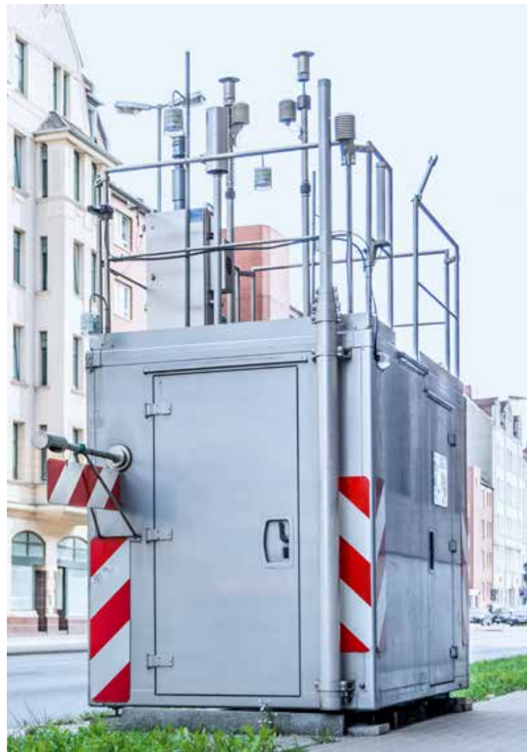
Measuring station for immission monitoring
